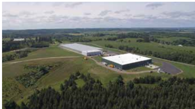
The 40,000 sq. ft. steel fish house and 123,000 sq. ft. glass greenhouse are situated on a 720-acre native restoration property in Northfield.
