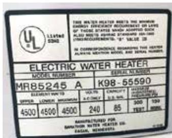
This is the sticker on the 85-gallon water heaters needed for warranty replacements. The 105 and 100-gallon water heater stickers are similar in appearance.
