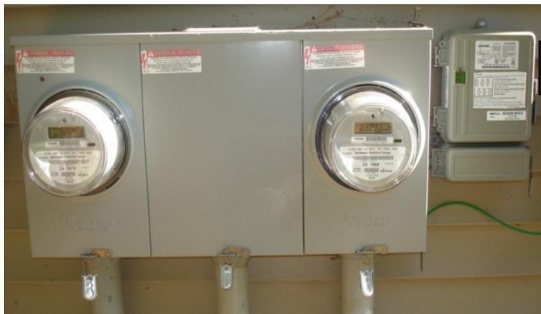
In most situations, your receiver is located outside near your meter socket. This photo displays two meters in which this residence is on the dual fuel program. If you are not a participant in the dual fuel program, you will only have one meter.
